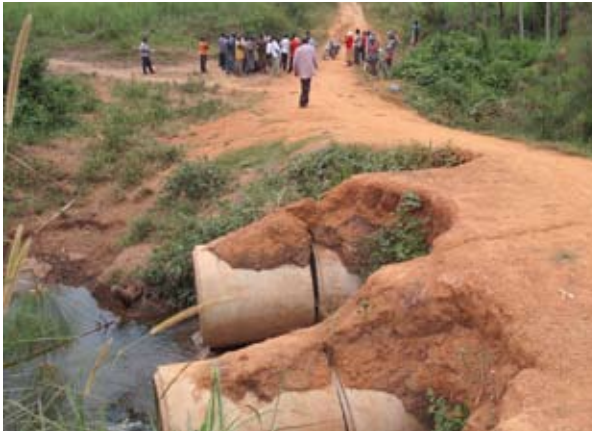
Ibuhe Bridge which broke down two weeks after construction in October 2010. The Bridge which connects several villages to Masindi –Butiaba road was subject of debate by Radio Kitara in Masindi
